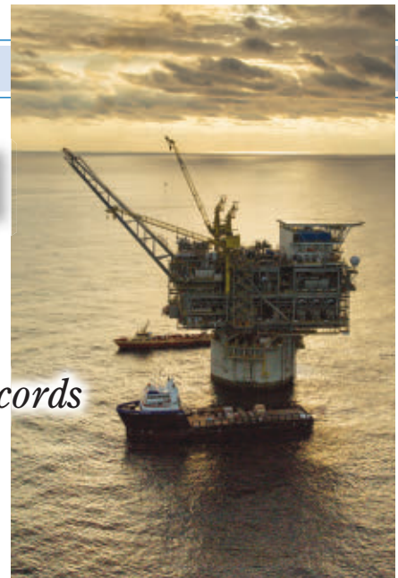
Anadarko's Lucius field and ExxonMobil's South Hadrian field produce through the Lucius truss spar. (Photo courtesy Anadarko Petroleum Corp.)
