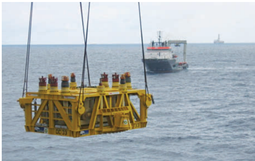
An FMC Technologies subsea manifold is lowered into the water as part of the development of Total's Egina field, located 150 km (~240 mi) off the coast of Nigeria. (Courtesy FMC Technologies, Inc.)
