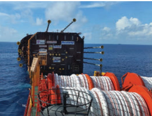
Pictured is the Heidelberg spar as it is being prepared for mooring work. (Photo courtesy InterMoor)
